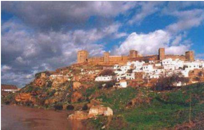
The Arab Castle in Alcalá de Guadaíra (Seville)
